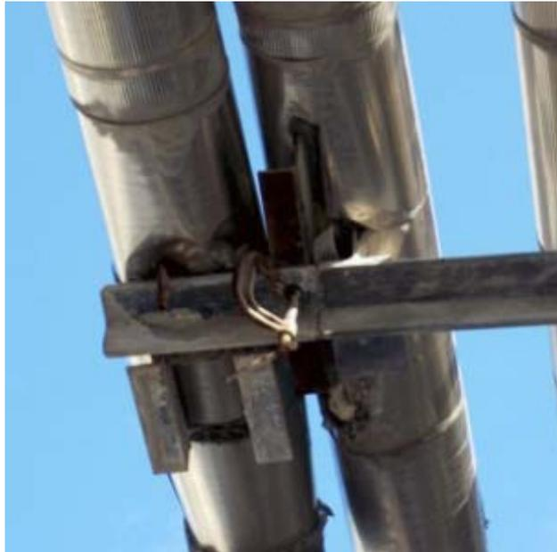
**Figure 2. Example of uncontrolled expansion and lack of guides to avoid buckling and lateral movement.**
