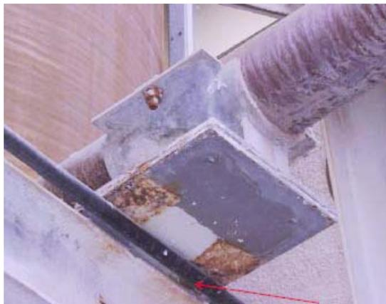
**Figure 3. Support at tipping point due to uncontrolled expansion.**
