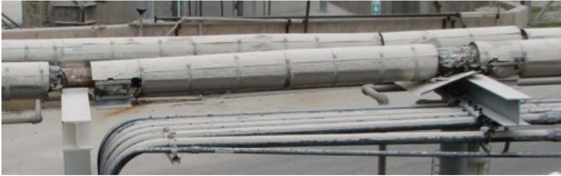
**Figure 1. Example of uncontrolled expansion.**
