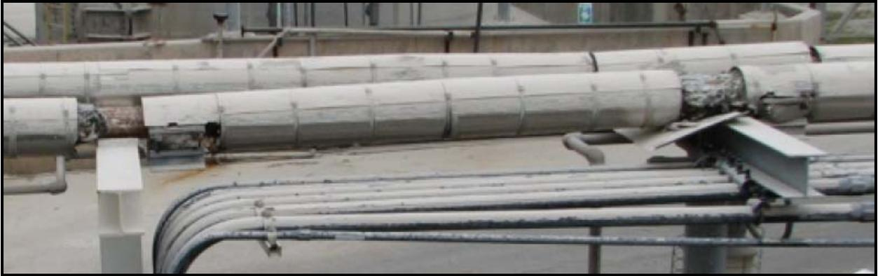
Excessive expansion has moved supports off of support steel and allows the pipe to be overstressed and damaged. Pipe has dropped 6"-7", insulation has been destroyed, and pipe rests on steel beam.
