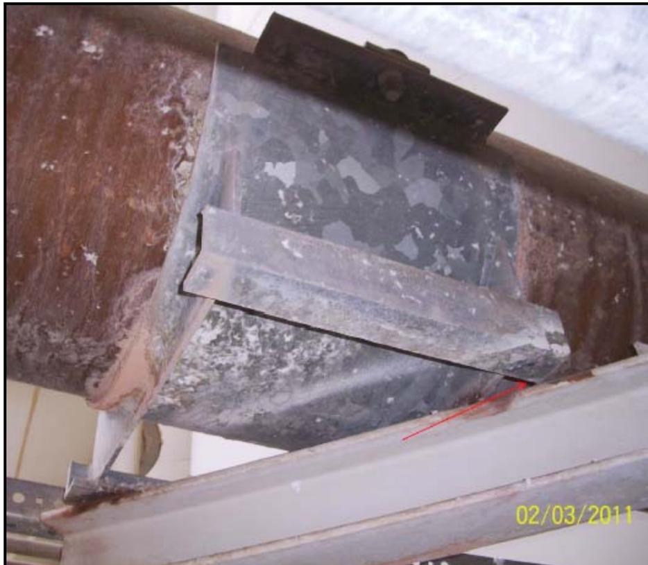
High local load and torsional moment (local stress) caused by tipped support.
