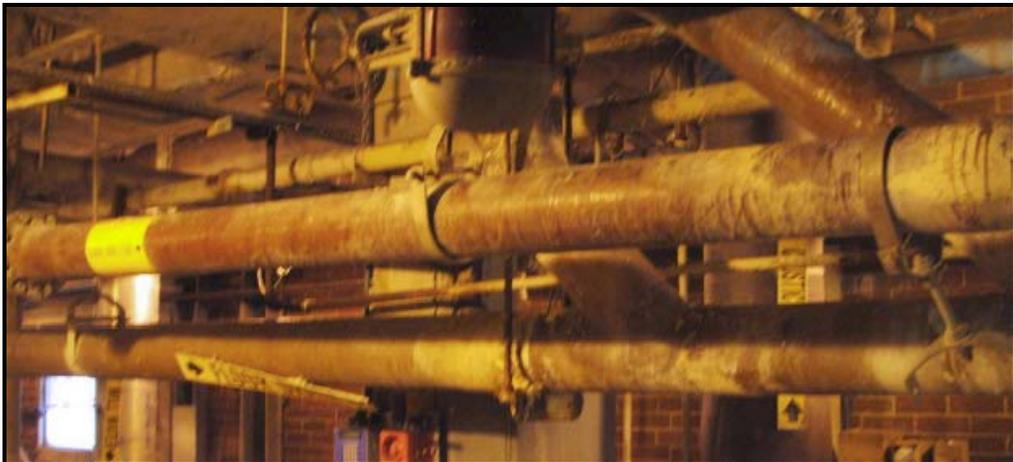
This photo depicts support failures that are caused by uncontrolled expansion and resulting over load and over stress. This entire process plant was designed without considering the effects of expansion and as a result the repair and pipe replacement have been continuous for more than 10 years since start up. The pipe is in such poor condition today only a complete replacement will solve the problem.
