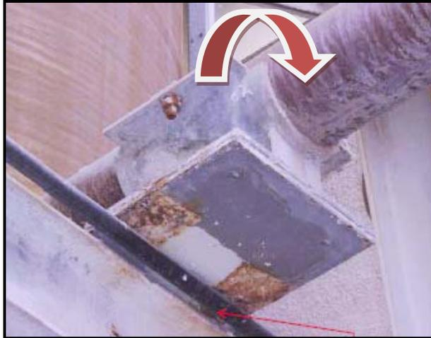
When the support moves off of the support steel a bending stress is added to the pipe.
