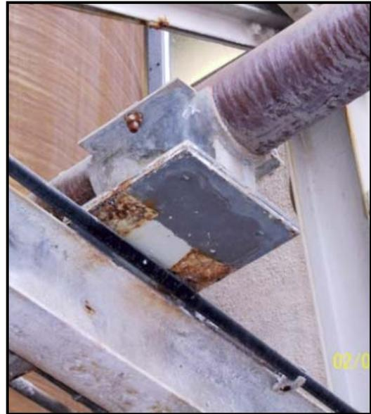
This is a typical condition throughout the process plant and the result has been a 15 to 20 year reduction in the service life of the FRP pipe. Maintenance has been constant since the plant was started more than 10 years ago.
