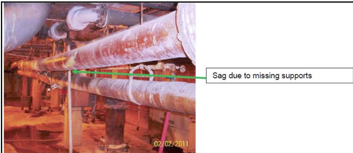
This process line has lost many of the clevis hangers due to excessive pipe expansion and results in severe overload of remaining hangers and high local stress on the pipe.
