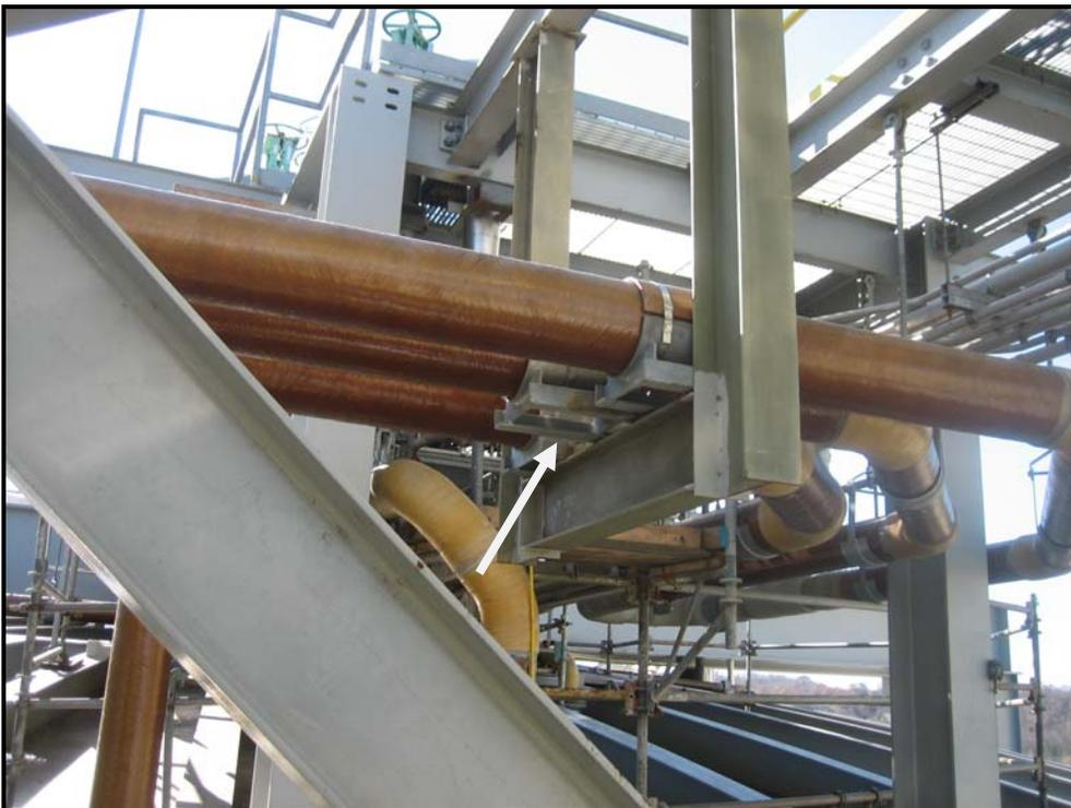
Uncontrolled pipe expansion - Supports moving off of support steel.
